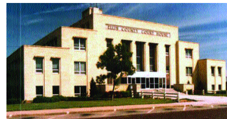
Ellis County Courthouse
